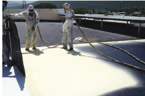
Spray in Progress
