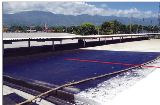
Roof was prepped on site
