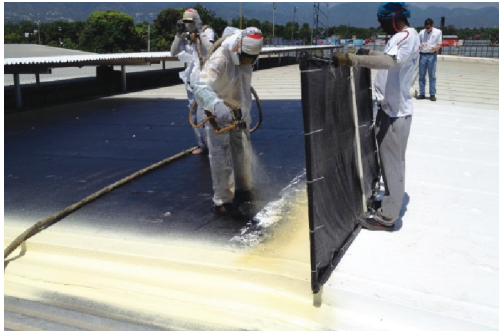
Spray in Progress
